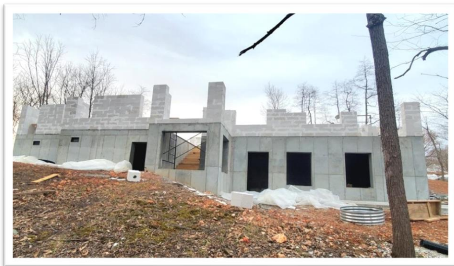
Figure 5: Concrete Foundation with AAC Block, Bentonville Arkansas
