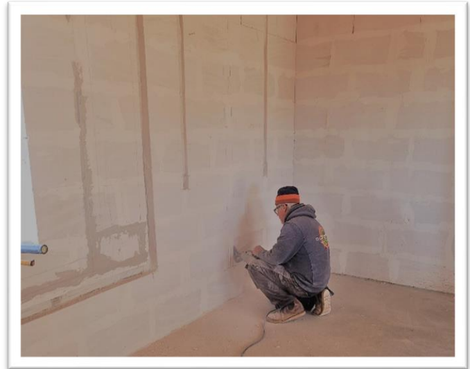
Figure 2: Worker routing out Rough-in Electrical and Plumbing
